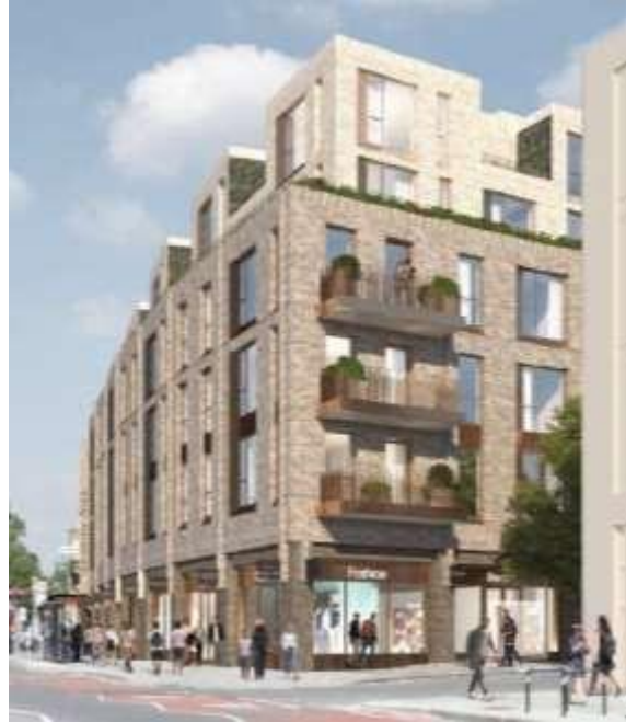
Figure 42: View of proposed Block C from the intersection of Denmark Hill and Orpheus Street.
